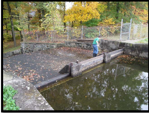
Primary Spillway with stop logs
